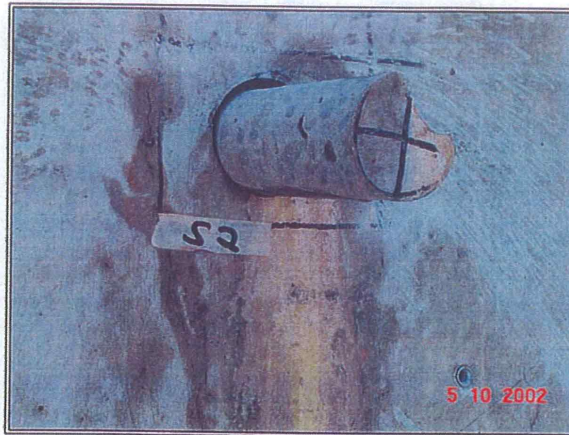
Core S2 was extracted at the tie pin on wall 1.
